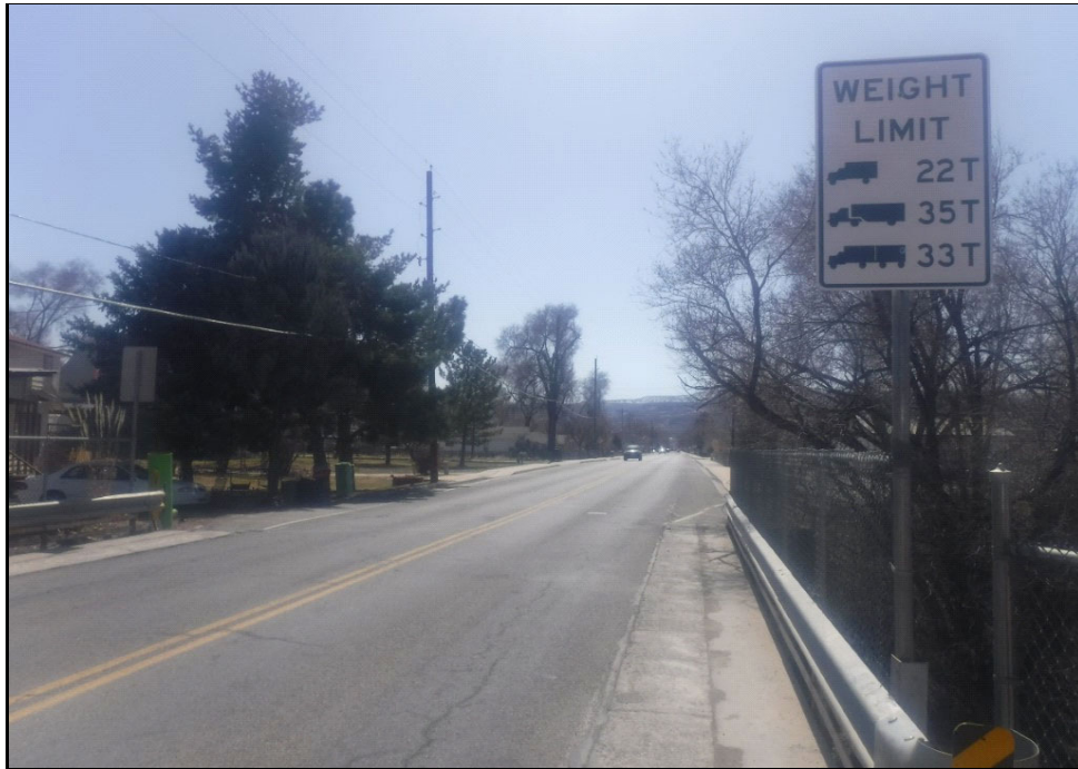
North approach load posting sign
