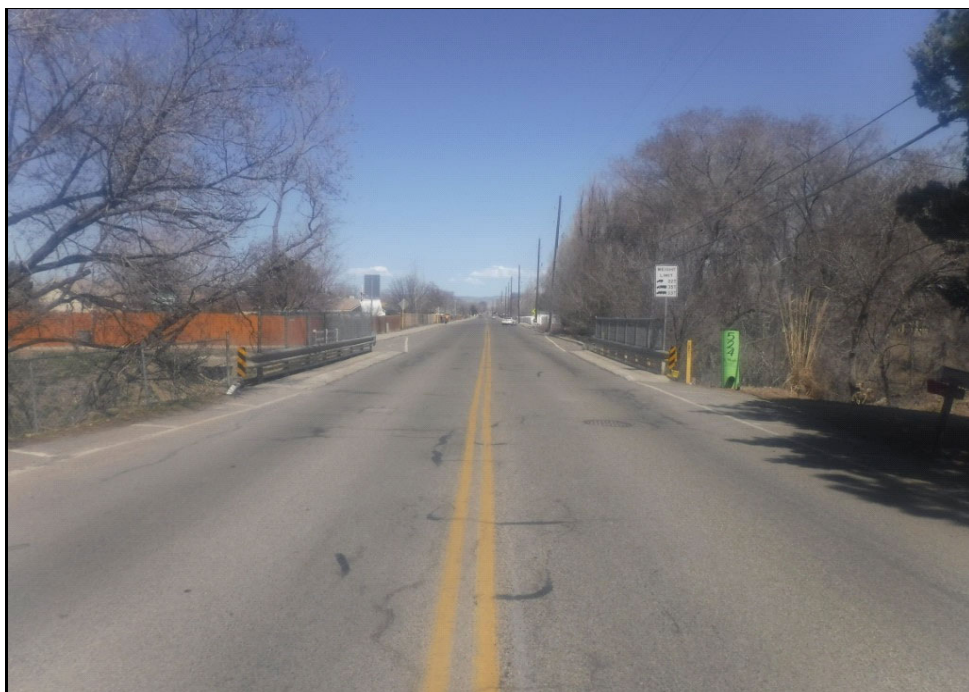
Roadway looking north
