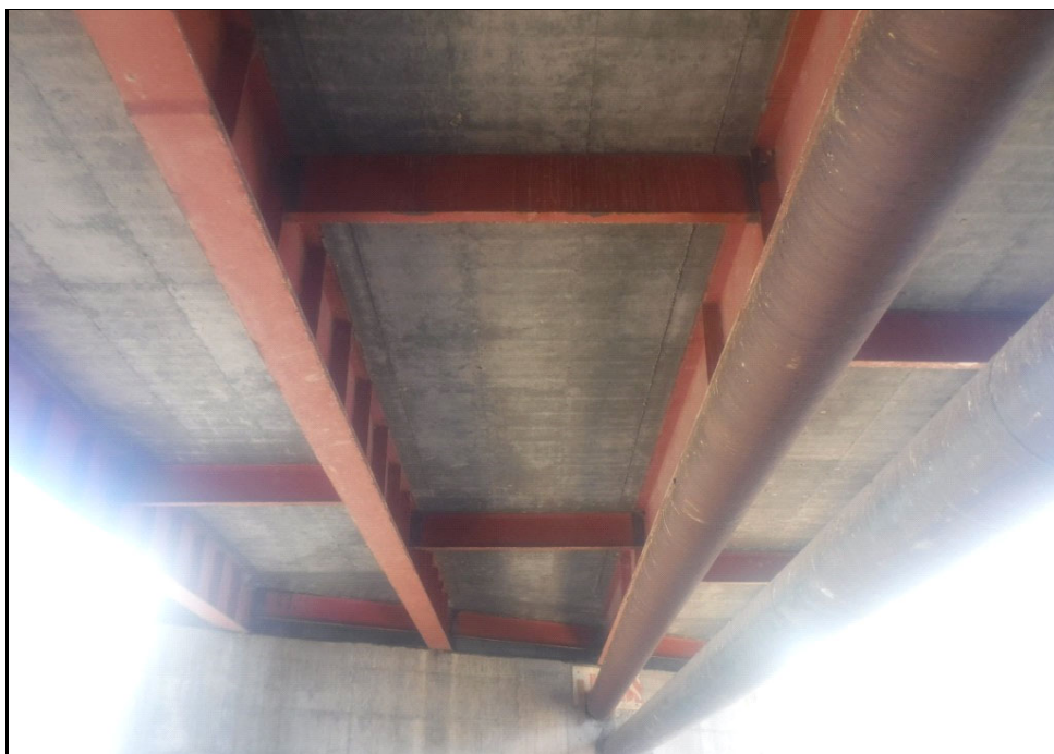
Superstructure looking north
