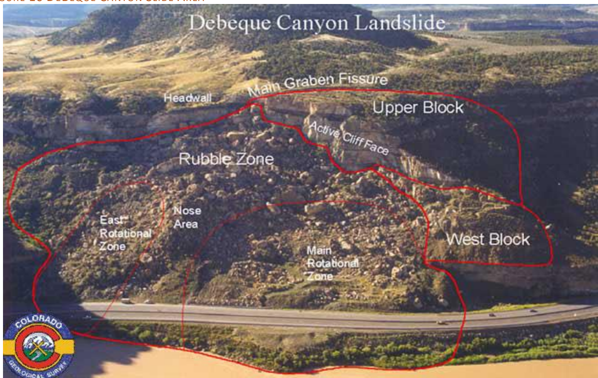
FIGURE 10 DEBEQUE CANYON SLIDE AREA
