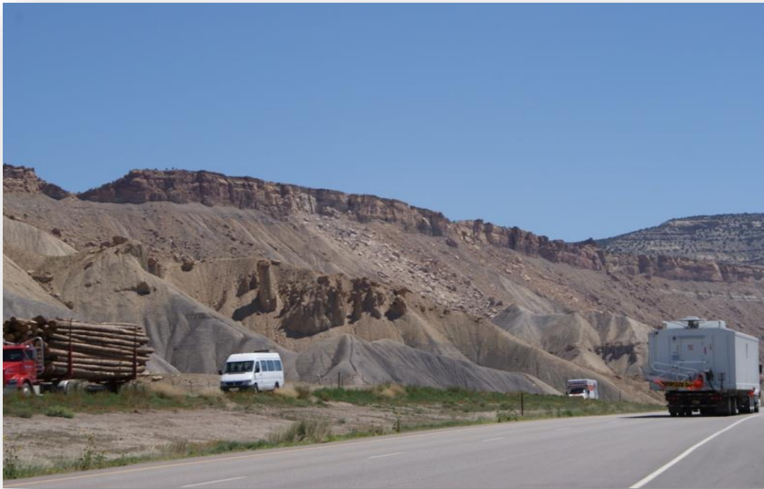
FIGURE 13 ROCKFALL WEST OF PALISADE ALONG INTERSTATE 70
