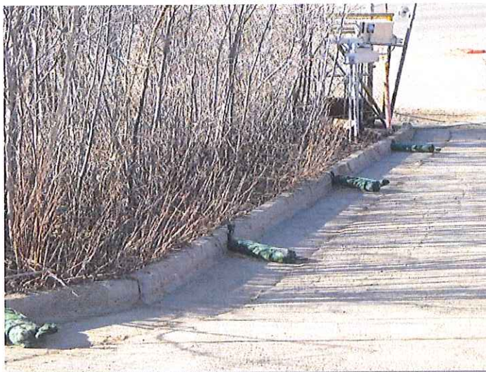
Photograph RS-1. Rock socks placed at regular intervals in a curb line can help reduce sediment loading to storm sewer inlets. Rock socks can also be used as perimeter controls.
