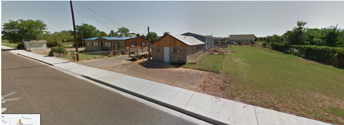
Street View of Property from 18 Road
