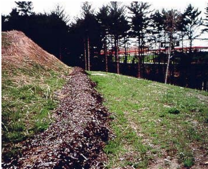
Photograph BB-1. Brush barrier constructed with chipped wood. Photo courtesy of EPA.
