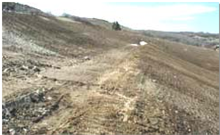
Photograph TER-1. Use of a terrace to reduce erosion by controlling slope length on a long, steep slope. Photo courtesy of Douglas County.
