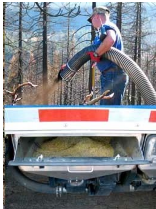
Photograph CB-1. Application of a compost blanket to a disturbed area. Photo courtesy of Caltrans.
