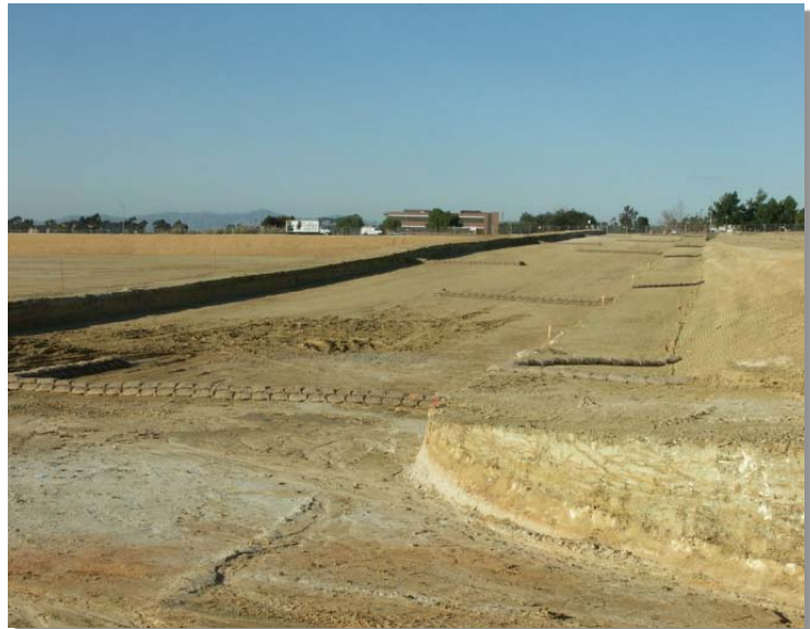
Photograph RCS-1. Rough cut street controls.
