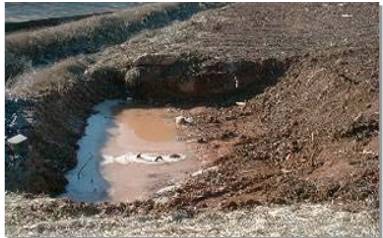
Photograph ST-1. Sediment traps are used to collect sediment-laden runoff from disturbed area. Photo courtesy of EPA Menu of BMPs.
