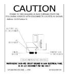
**Directory Placard: 705.10** — Where equipment is in multiple locations a directory placard shall be installed at each equipment location and at the location(s) of the system disconnect(s) and the layout must match the field conditions and the approved plans. This placard is to provide information as to where the array is located for first responders and to show the location of any load centers or other disconnection devices.
