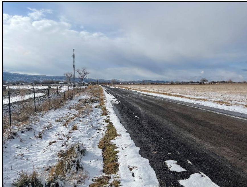
Image 4 – Looking West from the Project Access
