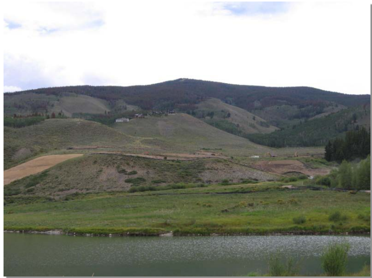
Photograph CP-1. Construction phasing to avoid disturbing the entire area at one time. Photo courtesy of WWE.
