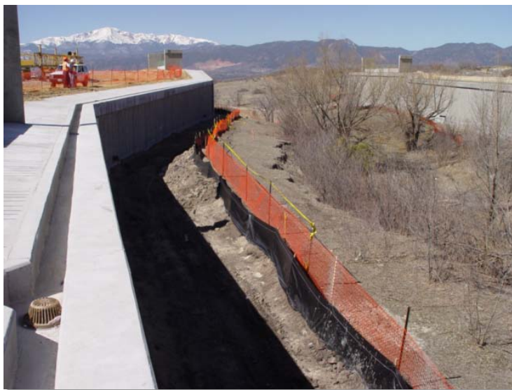
Photograph PV-1. Protection of existing vegetation and a sensitive area. Photo courtesy of CDOT.
