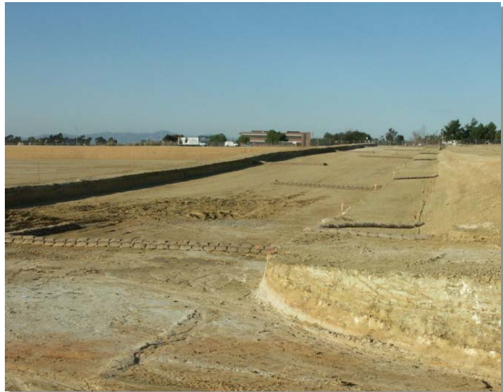
Photograph RCS-1. Rough cut street controls.
