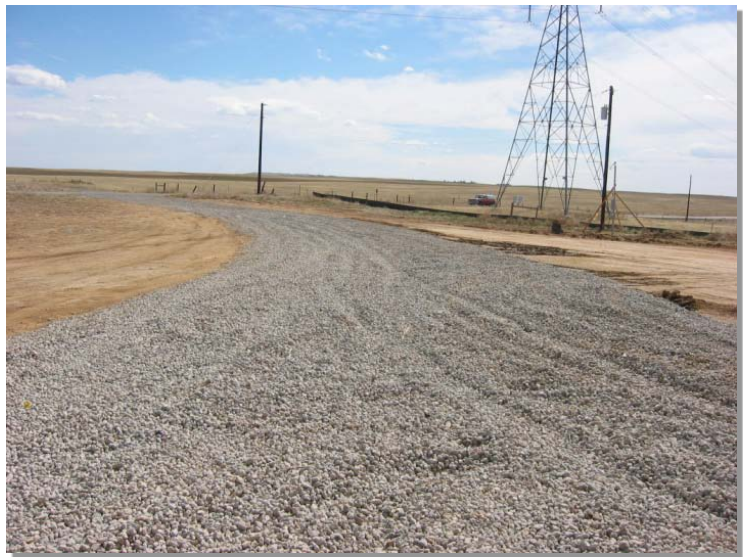
Photograph SCR-1. Stabilized construction roadway.
