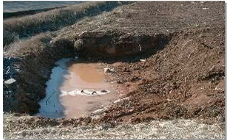
Photograph ST-1. Sediment traps are used to collect sediment-laden runoff from disturbed area. Photo courtesy of EPA Menu of BMPs.
