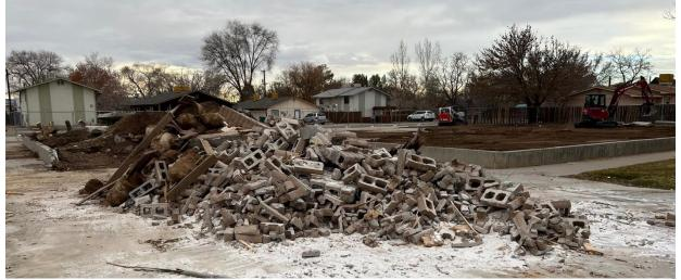
The contractor has started and is moving quickly with the demolition of facilities. The playground equipment, the restroom facility, playground safety material, horseshoe pits, and concrete surrounding the playground have been removed. The contractor will provide a 3-week schedule with upcoming work and that will be included in future updates, along with on <u>the project page</u>, and on social media.
