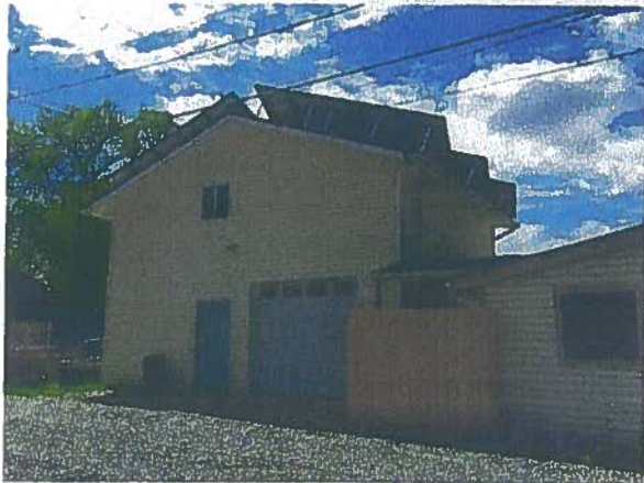
North & West sides of garage from alley
