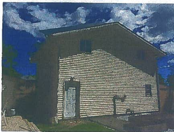
Entrance to ADU from yard, South side of garage
